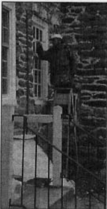
Ongoing restoration at Glen Fern.
