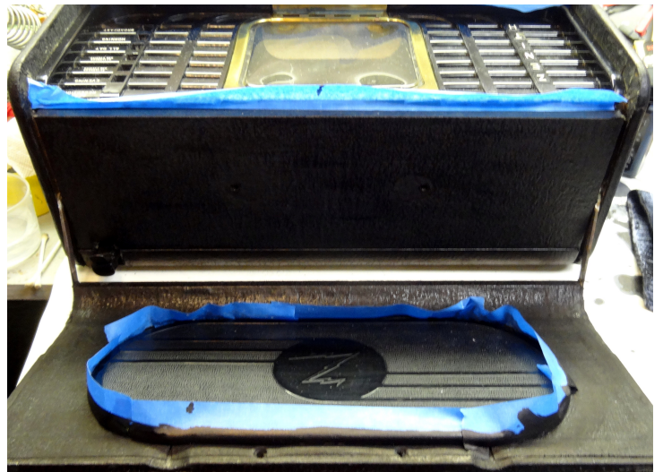
Carefully mask areas you do not want painted with the black leather dye. Cover the entire dial area also to avoid accidents.
