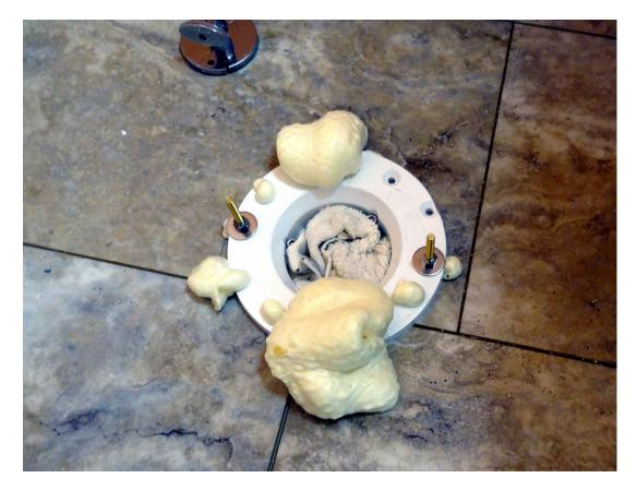
New flange extender in place and foamed. DO NOT touch the foam until it dries. It is then easy to break off. Before foaming I tightened the three flange bolts inside the new PVC piece.
