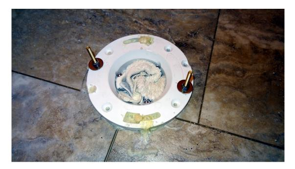
The completed flange ready for the toilet. You can see the three flange extender bolts which are tightened with a hex key. This makes for a very secure installation. If necessary it could be removed but not in my lifetime! The flange bolts are 3 ½ inches and no trimming of the length was necessary after installing the toilet.
