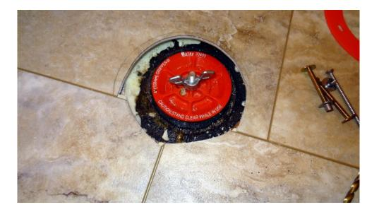
Photo of the old cast iron flange in good shape but 1 ¼ inches below floor level and not level to floor. The sub floor was cutout much bigger than this leaving gaps to the craw space. They were filled with foam around the edges. The top floor was further notched on each side to make clearance for the two flange bolts.
